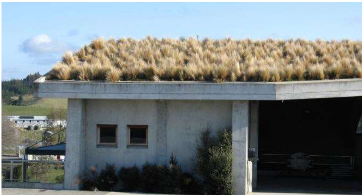
Figure 22: Tussock on roofs at Mahana Estate, Mapua.
