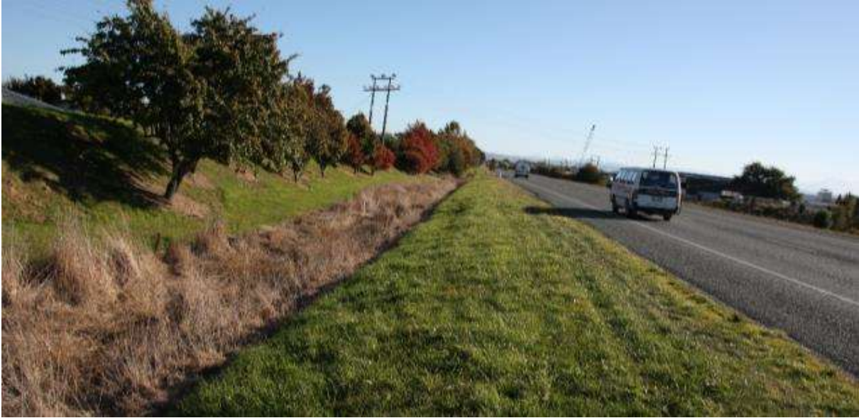
Figure 37: Highway swales, Richmond.
