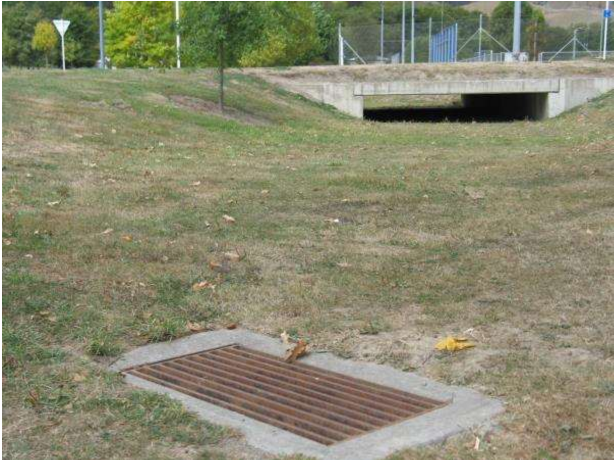
Figure 32: Saxton Field swale and overland flow path, 2011 (very short – usually minimum 100 mm height for swales – discuss with Parks implementing different mowing standards within playing grounds, including potential for planting up).
