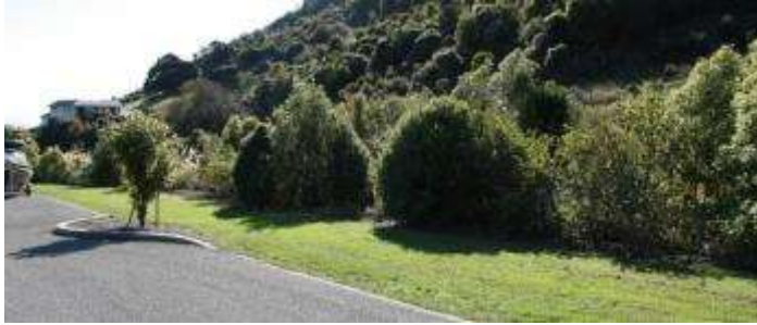
Figure 14: Filter strip: Saddleback Road, Todds Valley with street tree located for efficient maintenance and protection from mowers.
