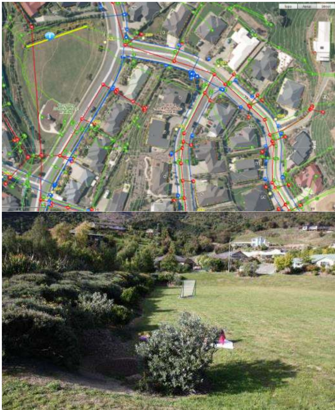
Figure 26: Frenchay Drive Playground – dry pond.
