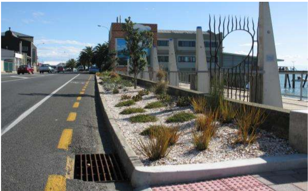
Figure 43: Port Nelson 2011 – this should be receiving runoff from footpath if not the road, which would benefit tree health and trap coarse litter.
