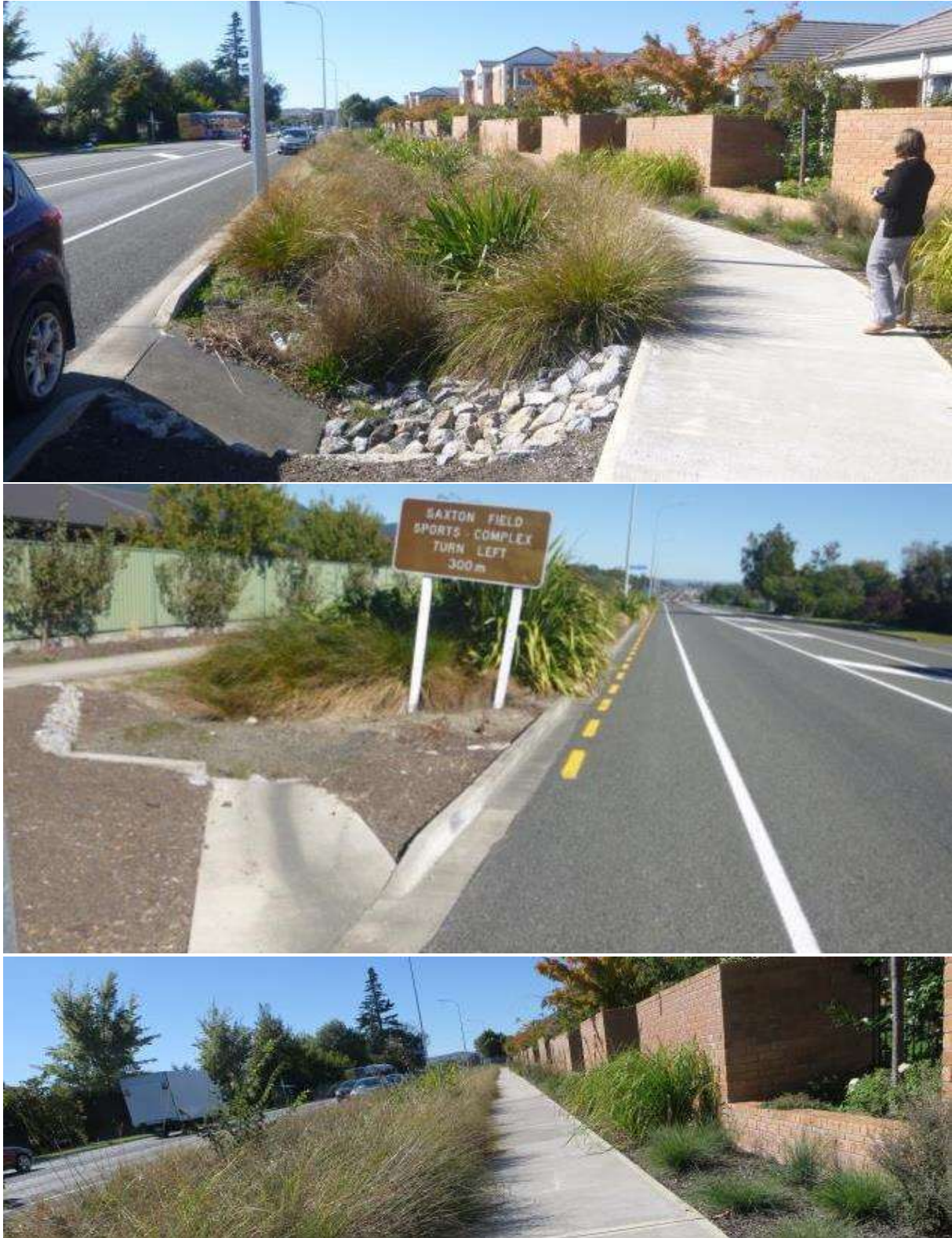
Figure 34: Main Road Stoke swale.
