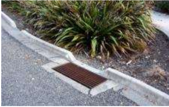
Figure 5: A design defect kerb inlet just before inlet to device.
