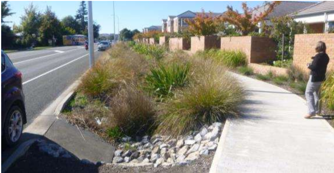
Figure 4. Planted swale on high-capacity road in Stoke (April 2016). The dense cover of native sedges and small flaxes avoids the traffic disruption of frequent mowing and is a more effective buffer against traffic for pedestrians.
