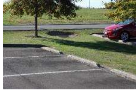
Figure 15: Swales at aquatic centre, Richmond.
