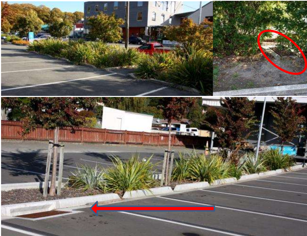
Figure 28: NMIT bioretention; the circle shows the overflow height which allows only minimal ponding depth; the arrow shows how runoff can bypass the swale directly to the catchpit.
