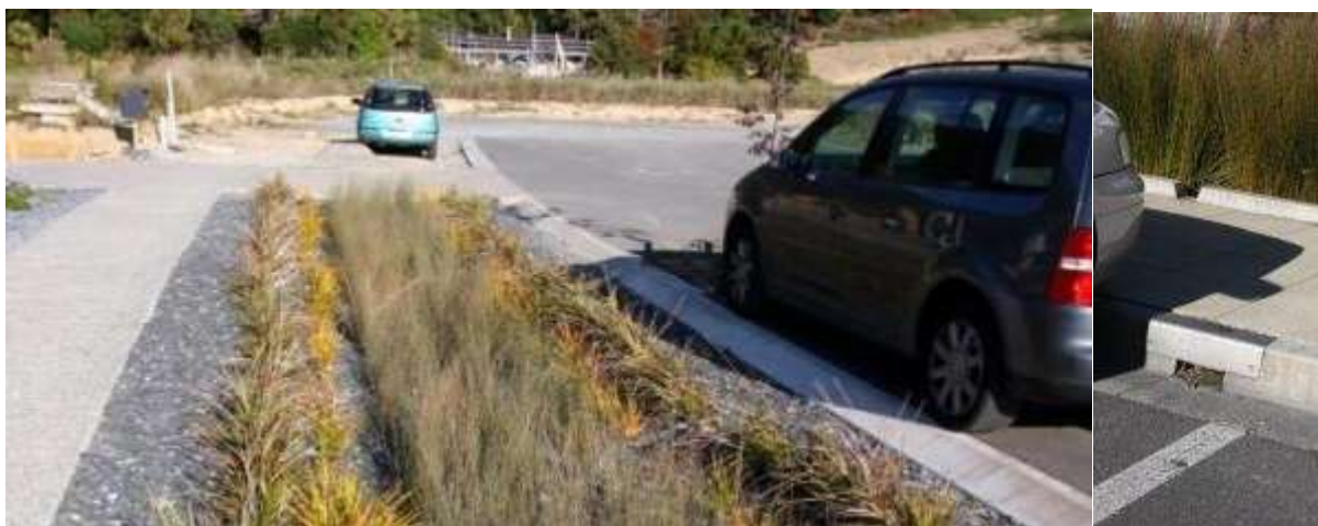
Figure 17: Bioswale in Sanctuary Drive (left photo). Raingarden in Sundial Square has attractive planting but the small, narrow inlets are prone to blocking and difficult to maintain (Right photo).
