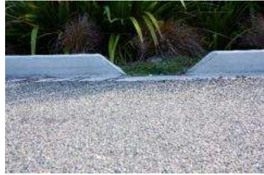
Figure 6: A construction defect. Ground level in device higher than surrounding hard surfaces impeding inflow.
