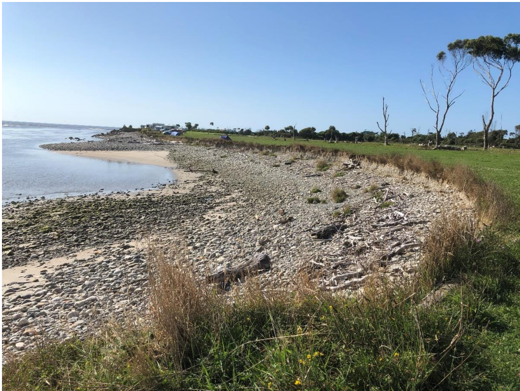
Figure 3-3: View seaward on north bank, showing relatively recent erosion "bite" into cobbly terrace fronted by cobble lag beach.
