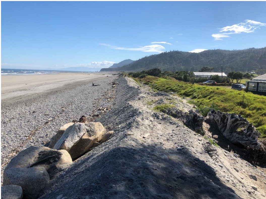
Figure 3-5: Double bund fronting Mokihinui township. Note steep (at angle-of-repose) seaward face of seaward bund, cobble ramp on upper foreshore, and wide sandy lower foreshore.
