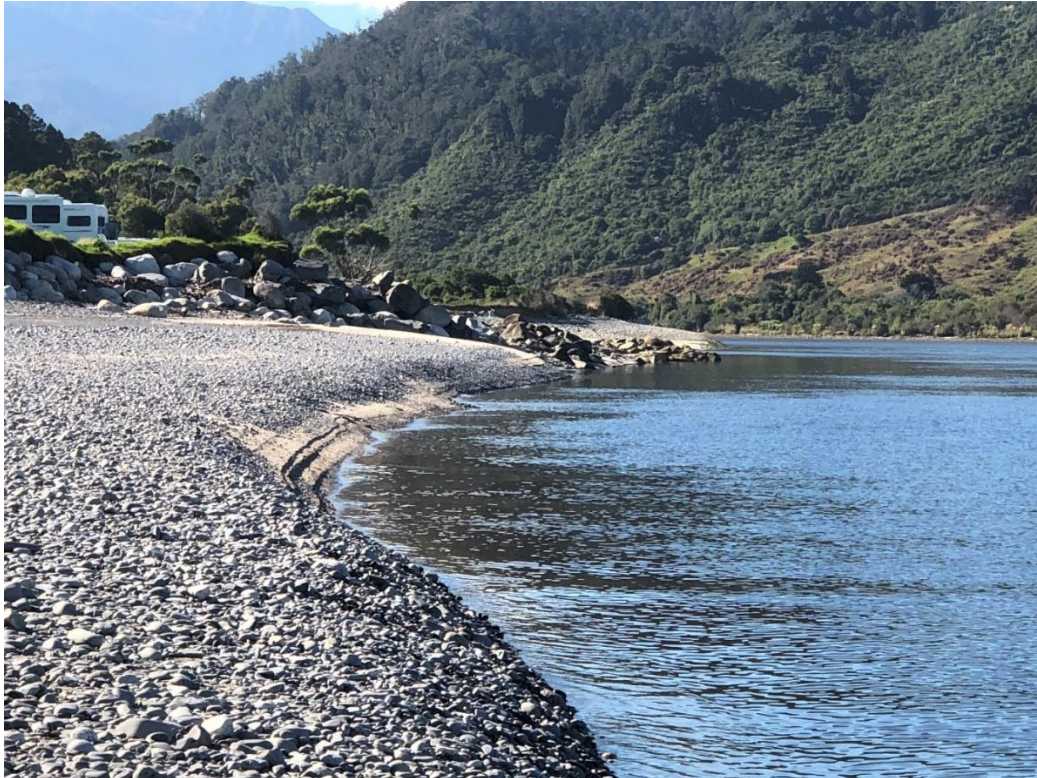
Figure 3-1: View upstream on north bank to the root of the training wall. Rock riprap in front of campervans has partially collapsed.
