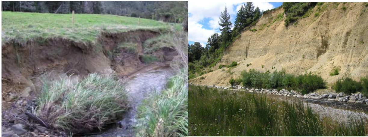
Figure A1.5. Examples of streambank erosion. (Left) mass failure in fine alluvium caused by stream undercutting (Photo: Chris Phillips). (Right) streambank and cliff erosion (Photo: Chris Phillips).
