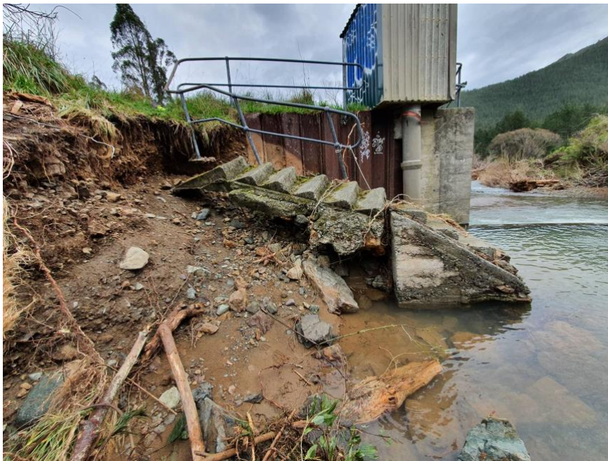
Figure 2: Scour and bank erosion. Photo by permission NCC
