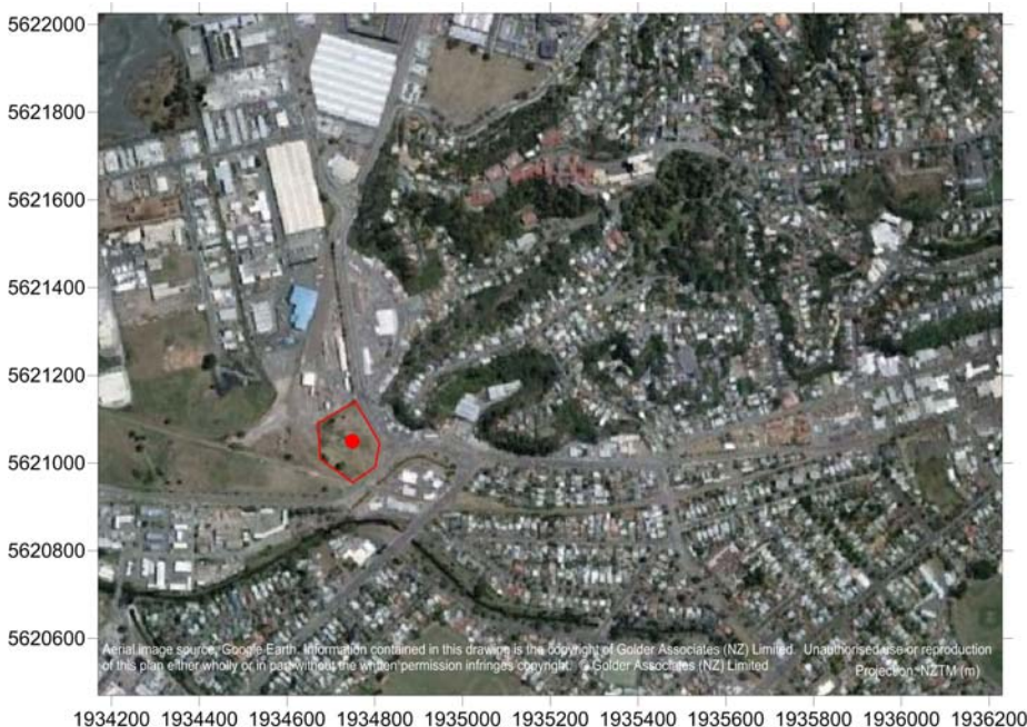
Figure 2: Aerial view of the location of the wood-fired boiler, Onekawa industrial area, Napier. Axes are in metres, in NZTM coordinates.
