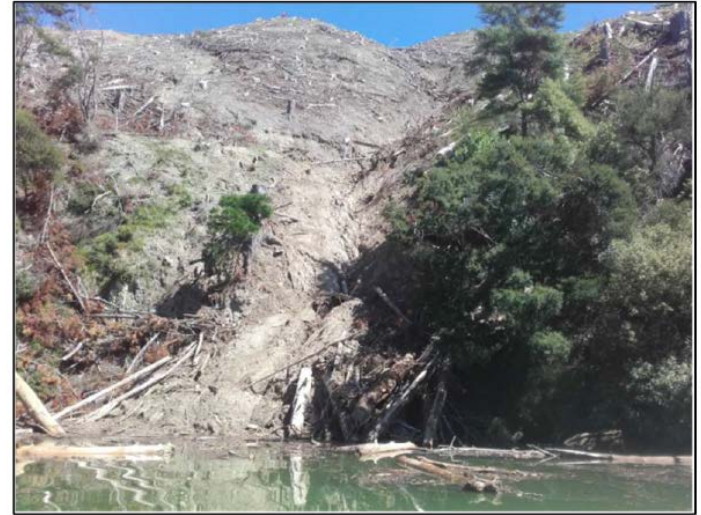
Figure 4.1: Failure in Whataroa Bay (February 2018).
