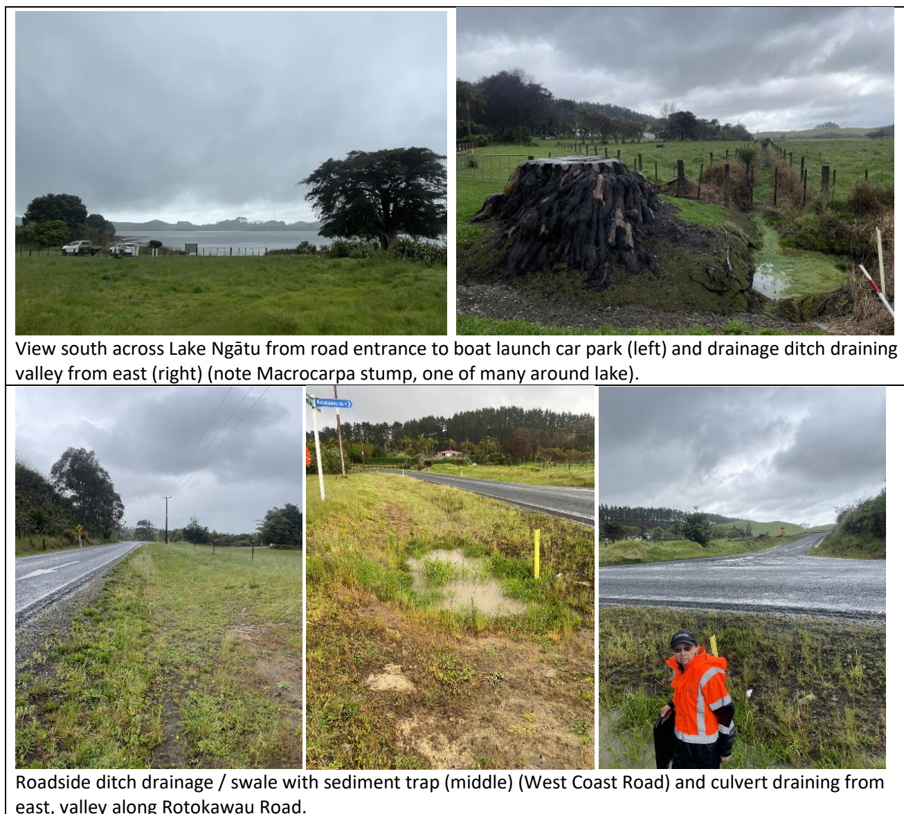
Figure A-1: Site 1: Carpark at boat launch area, drainage from Rotokawau Road and sediment trap.
