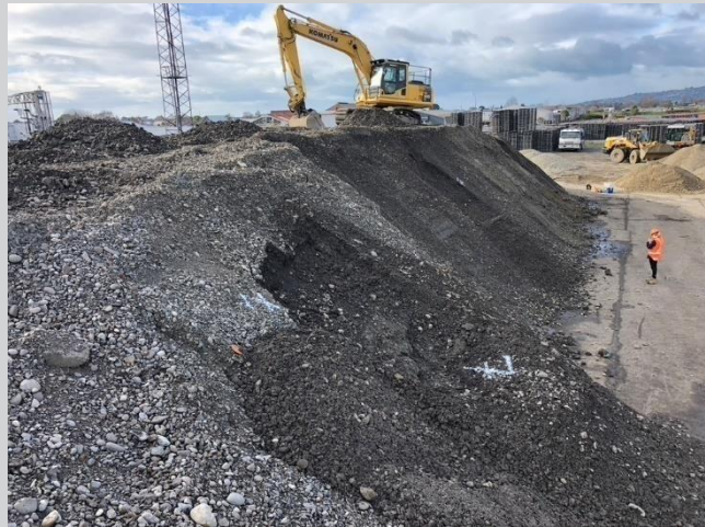
Stockpile of material generated through works
