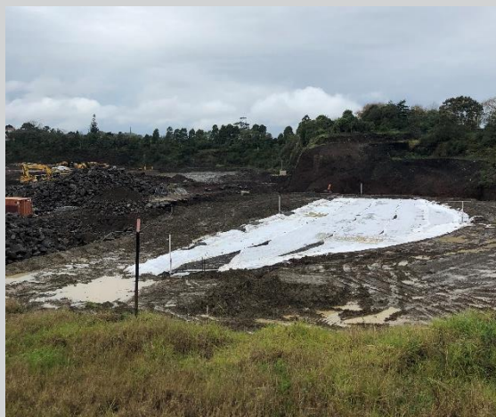
Reused, engineered surplus soil material in place
