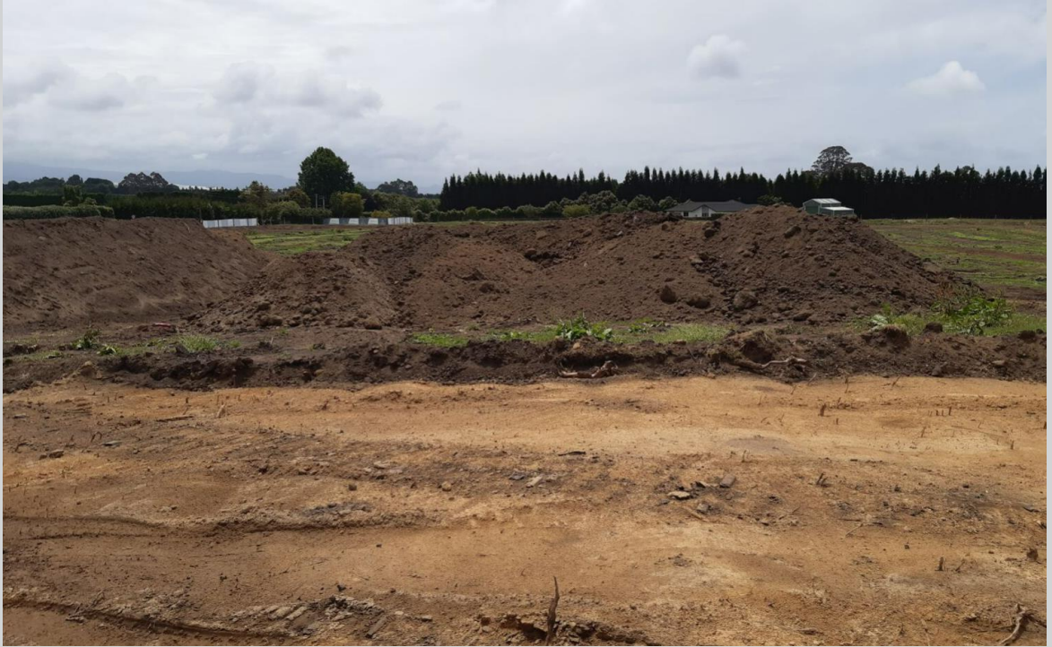
Ex-situ stockpiles of blended soils. (Case study provided by Richard Griffiths, Aurecon)
