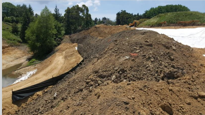
Encapsulation of asbestos-containing materials
