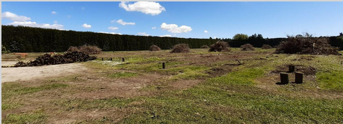
Initial site investigations showing presence of treated timber posts
