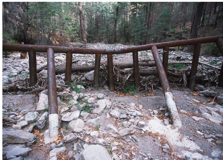
Figure 23: A more substantial debris catcher ('Slash Rack') installed in a higher risk catchment (Photo retrieved from USDA NRCS)
