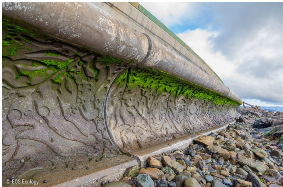
Figure A3.18. Curved textured seawalls constructed with precast concrete panels, as seen after installation.
