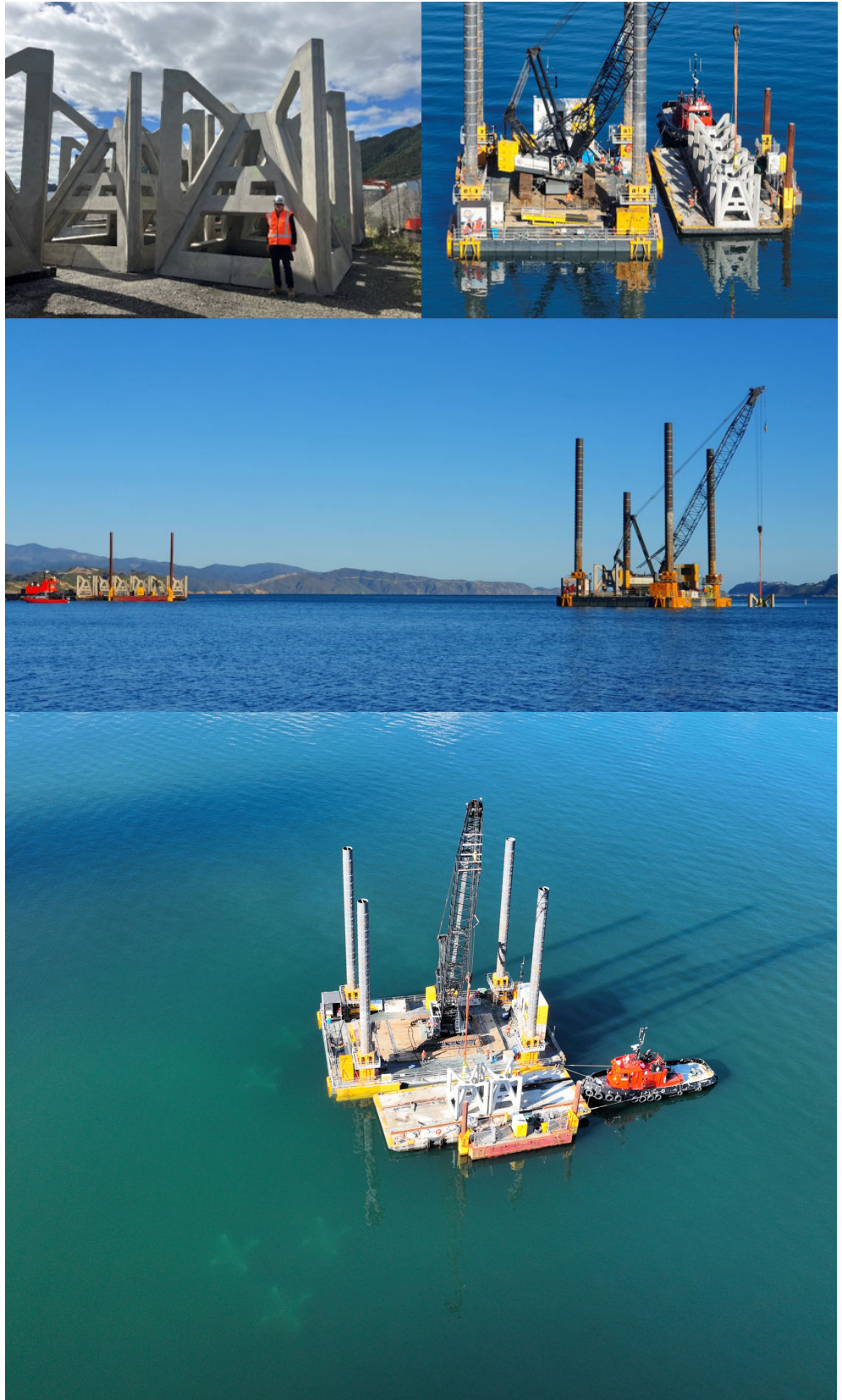
Figure A3.11. Reef unit fabrication and deployment
