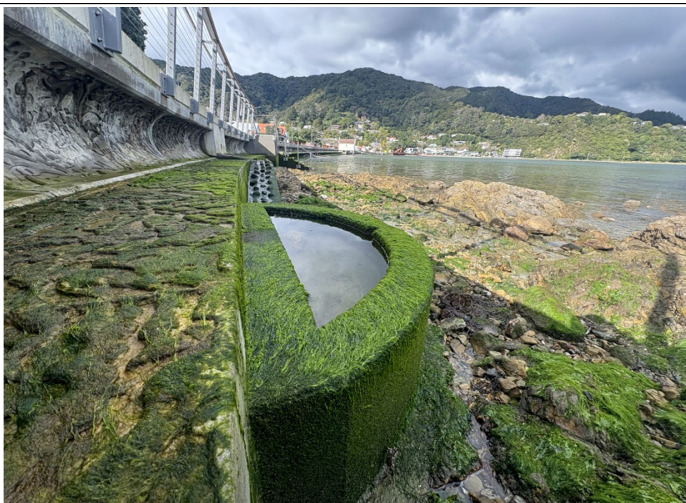
Figure A3.21. Constructed tide pools, attached to the finished seawall using a precast design made from concrete.
