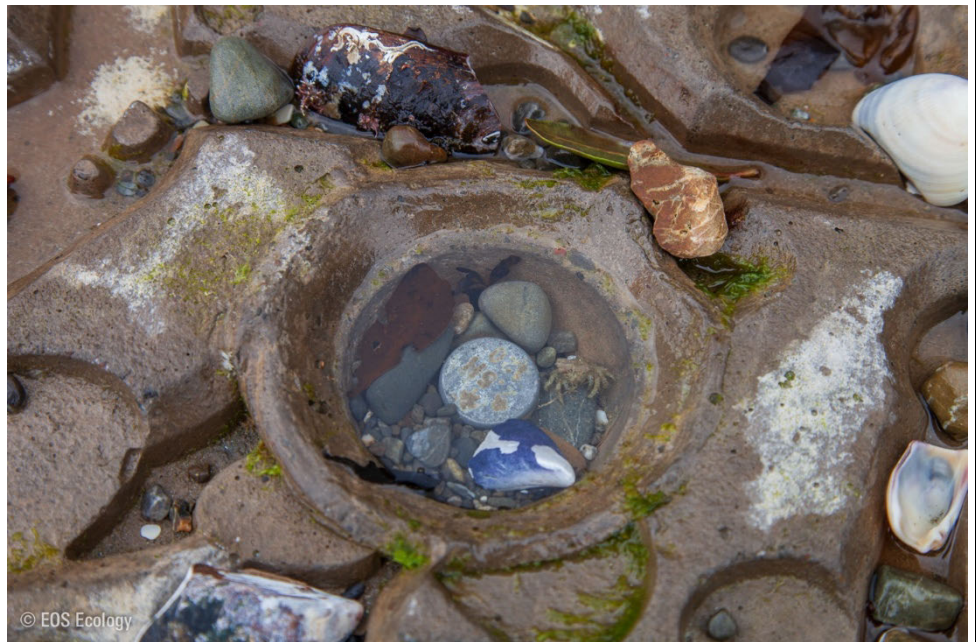
Figure A3.20. Small pools cast into the horizontal steps of the seawall.
