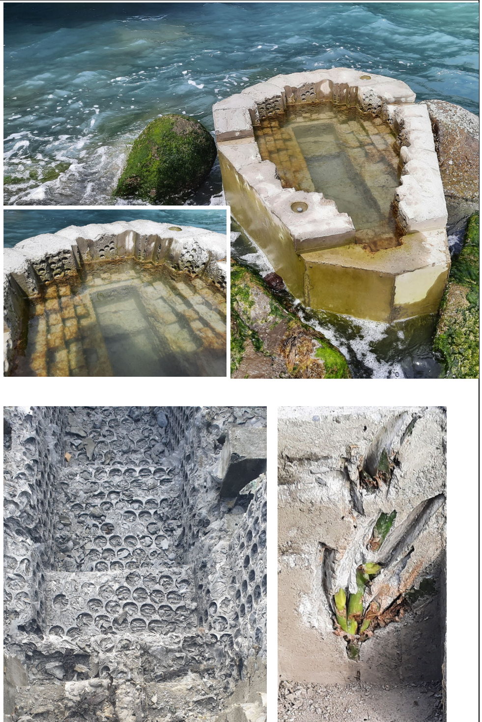
Figure A3.27. Top: One of the pools installed at Lyttelton Port, with a close-up view of the inside basin in the insert. Bottom: Details of the concrete texturing.
