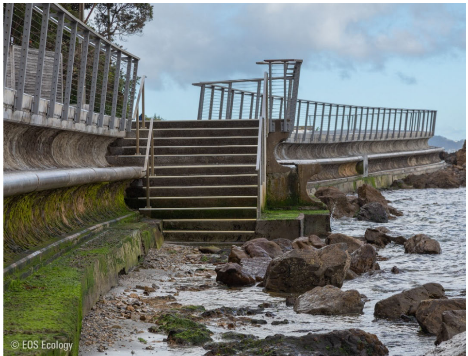
Figure A3.26. Stairs have been placed at key locations along the seawall, allowing the public to access the coastal area and engage with the intertidal zone while minimising encroachment into the coastal marine area.
