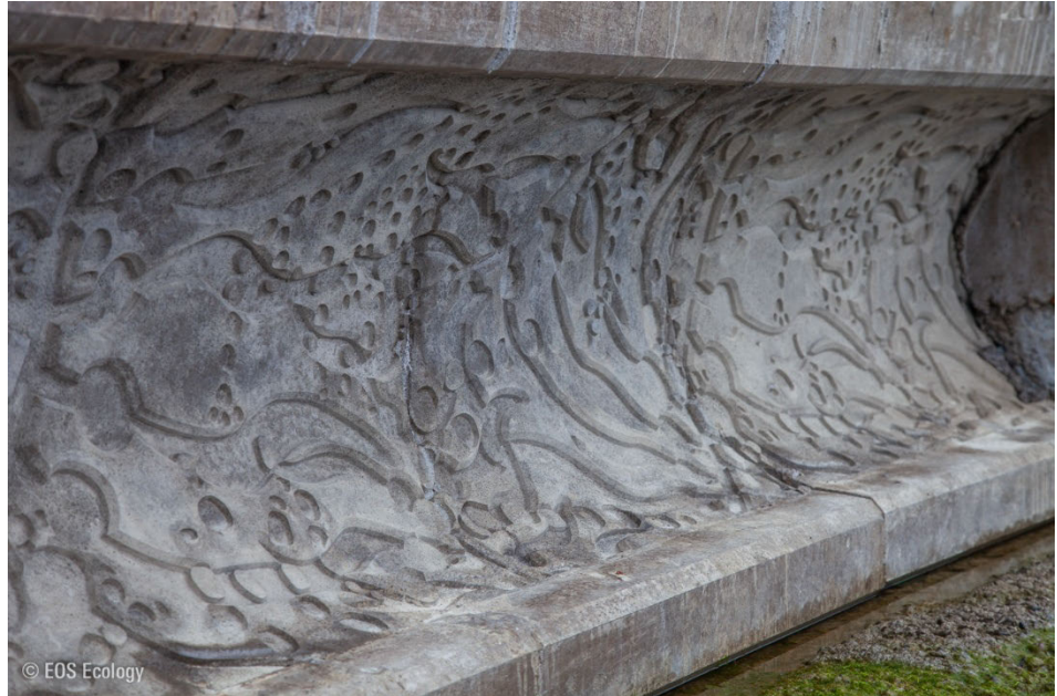
Figure A3.17. Curved textured seawalls constructed with precast concrete panels, as seen after installation.
