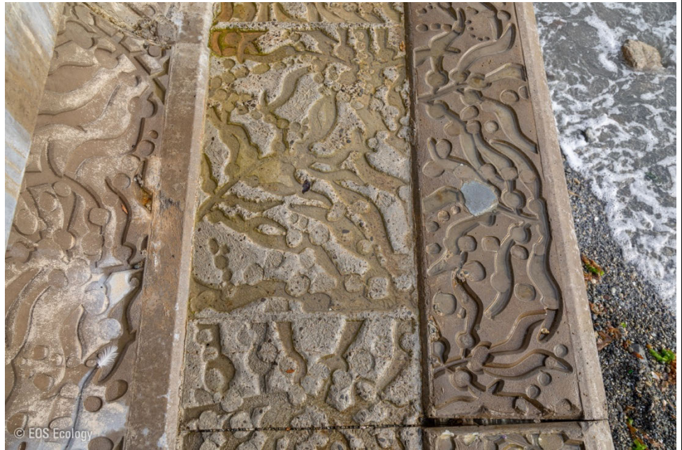
Figure A3.19. Horizontal platform between curved sections of the seawall, with precast concrete panels on the sides and a central panel of poured concrete stamped with the texture in situ .
